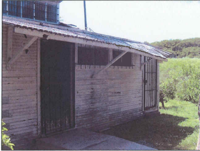
Front View of Frame House (No contributory value)
