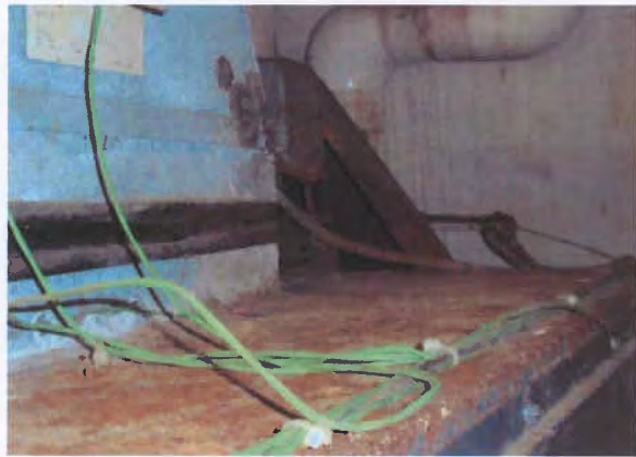
Figure 2 – Degradation of AHU Casing and Ductwork
