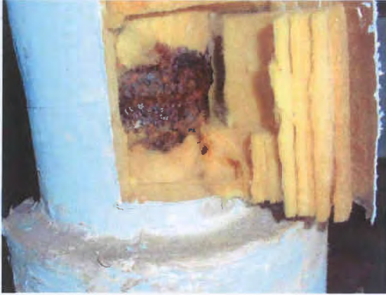
Figure 7 – Chilled Water Piping Condition Under Insulation
