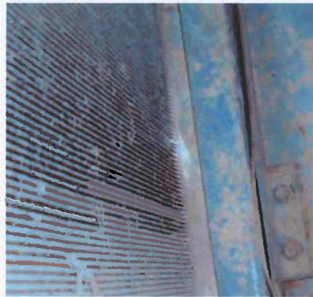
Figure 2 – Degradation of AHU Casing and Ductwork
